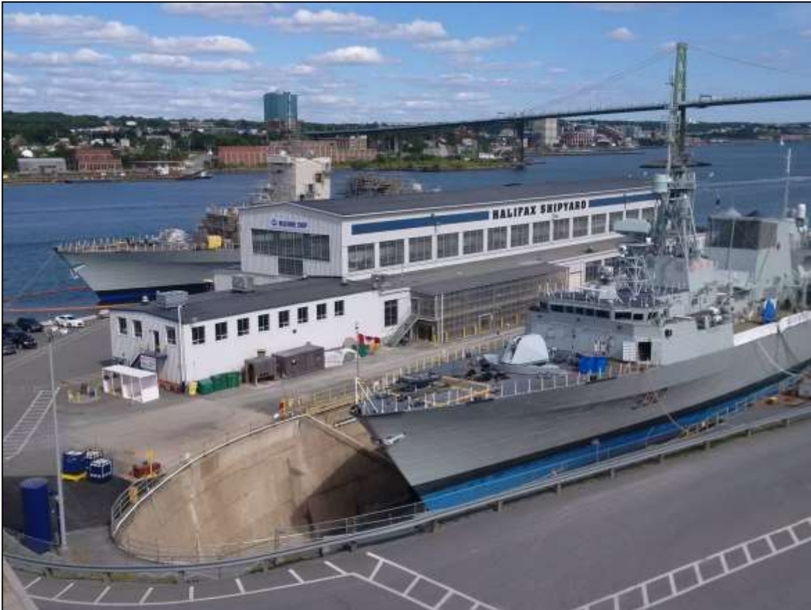
The Halifax Graving Dock in 2017 showing HMCS Ville de Quebec in the dry dock
