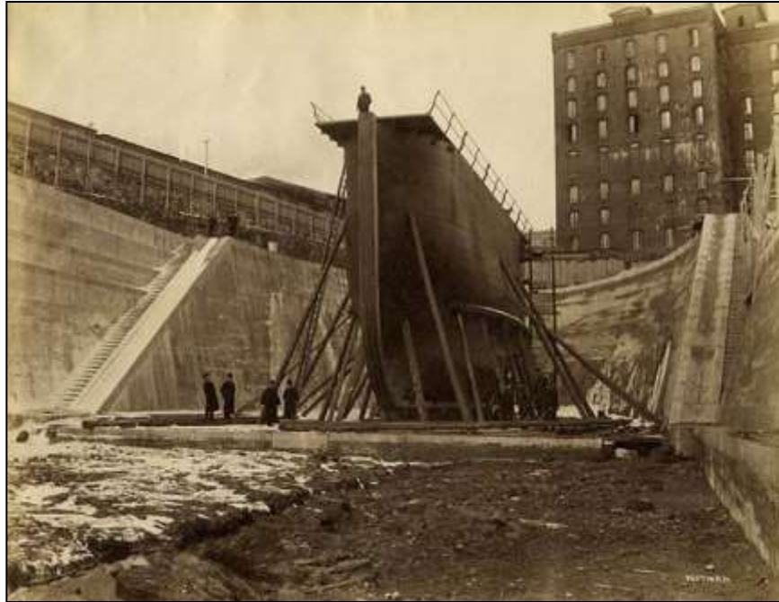
The caisson or gate for the Halifax Graving Dock being assembled within the dock itself circa 1888-89
