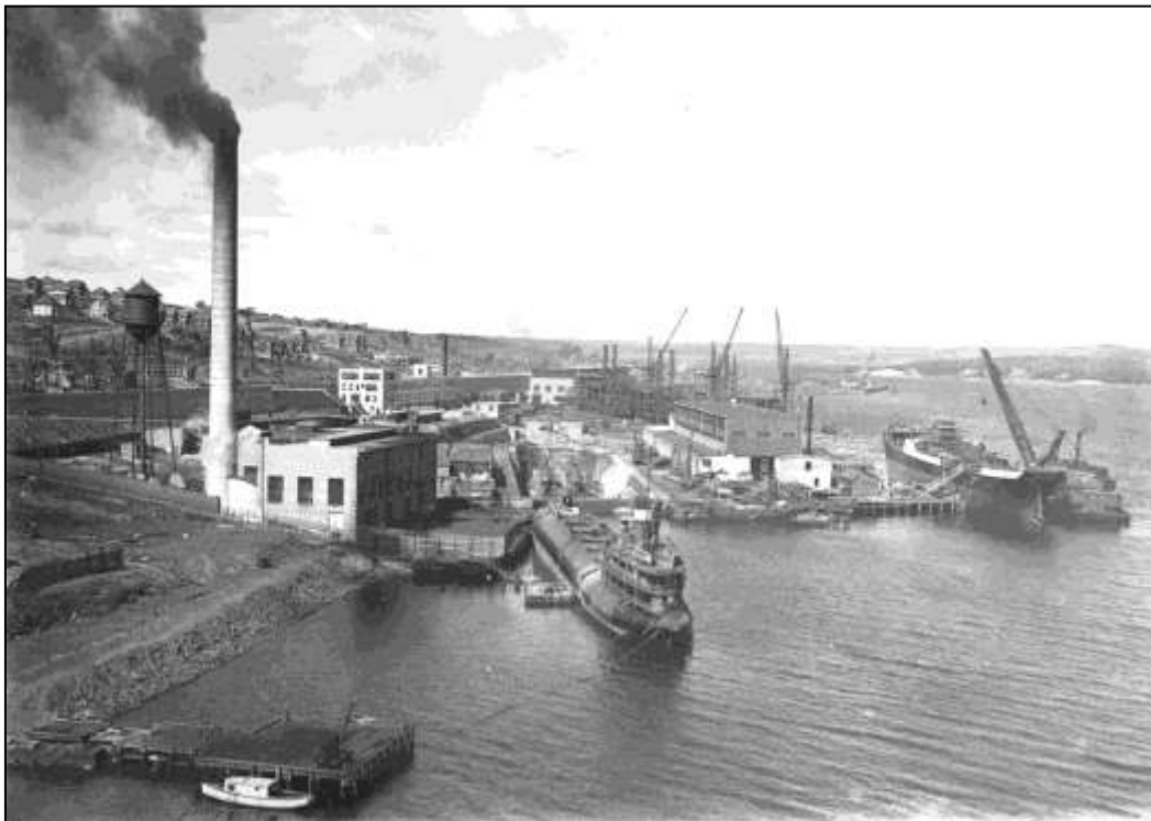
The Halifax Shipyard in 1920, having been rebuilt after the Explosion. Submarines CH-14 and CH-15 are shown in the Graving Dock, SS Canadian Mariner is alongside the Machine Shop wharf, and the whaleback barge Atikokan is in the foreground. The new building slips can be seen just behind the Machine Shop.
