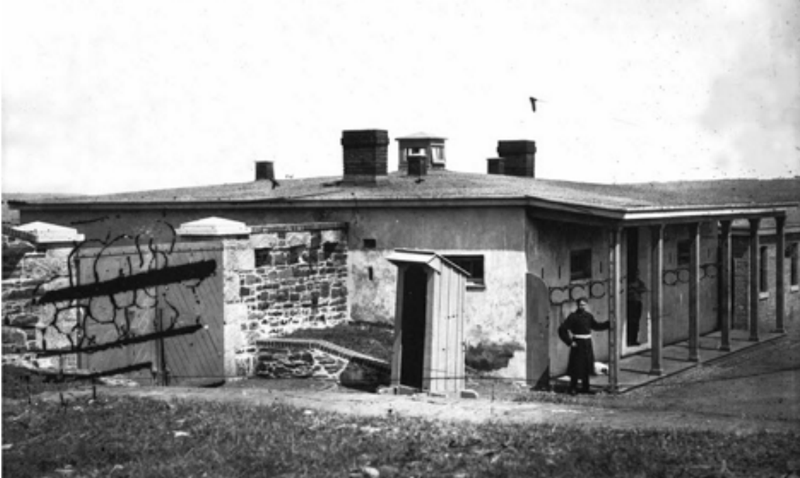
Piers' notes: No. 229. Ogilvie, Fort: Gate and Caponier (loopholed Barracks for twelve men and one N.C.O., and Guard Room) with piece of loopholed Wall at left; Artillery Store at extreme right; from inside the Fort; 1879(?). Looking North, from Southwest end of the fort. Prints of photographs of Fort Ogilvie are attached to Record Plan dated 1879.
