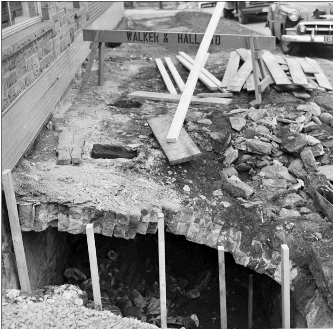
Figure 3.2-26: Vaulted storage rom under the sidewalk of Queen Street at the corner of Morris Street, encountered during construction activity in the mid 20th century, looking north towards Spring Garden Road. 104
