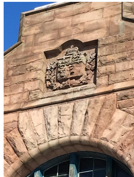
Detail at top of west wall
