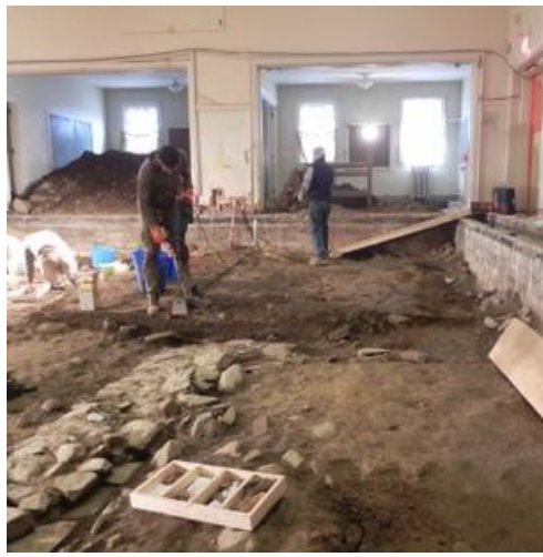
Colin Hicks operates an electric jackhammer to remove some of the heavily compacted soil that could not be managed with sma...
