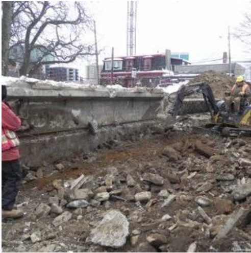
After demolition of the superstructure, April MacIntyre monitors excavations to remove the 1951 building foundations, which were...
